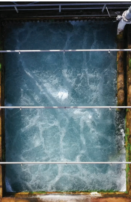
Water purification tank.
